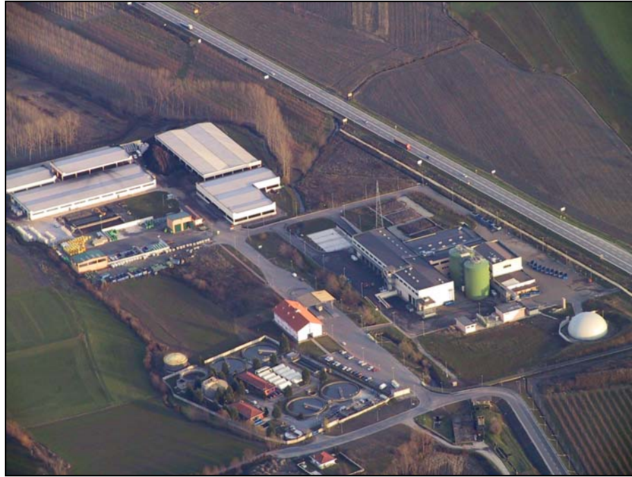
Figure 1. ACEA Waste treatment facilities, Pinerolo Ecologic district
